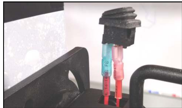
Fig. 9 (Red Wires to Switch)
